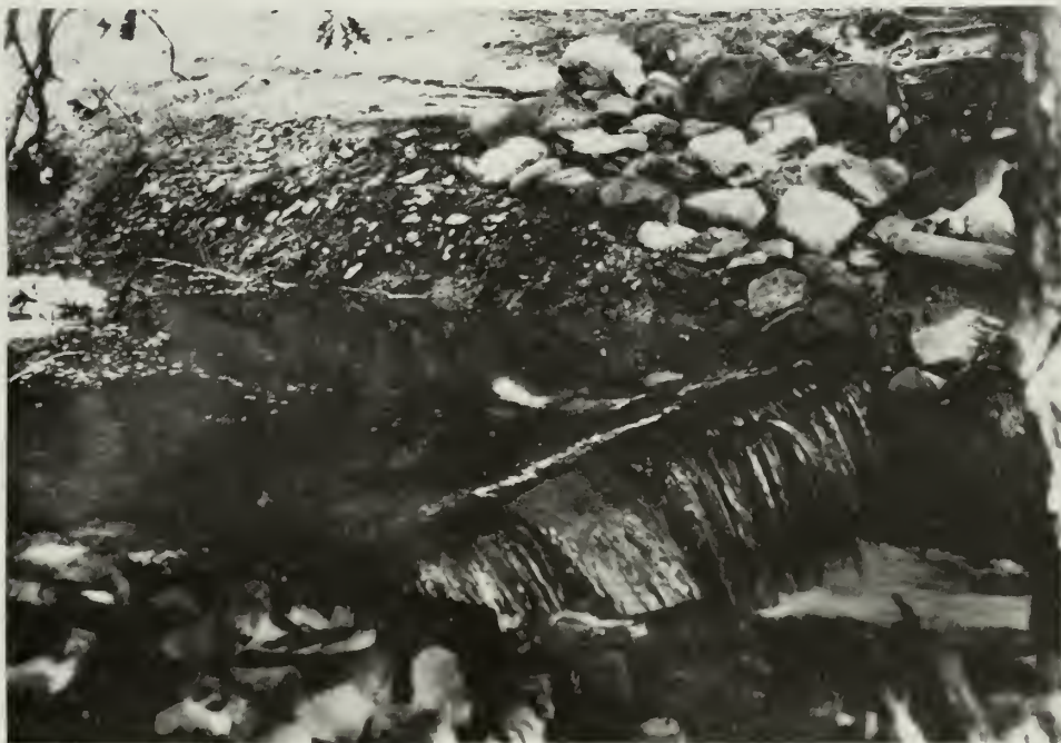
Figure 3.—Log stream improve structures such as this shown on McKnight Creek, New Mexico were first installed in the West in the 1930s by Civilian Conservation Corps workers.
