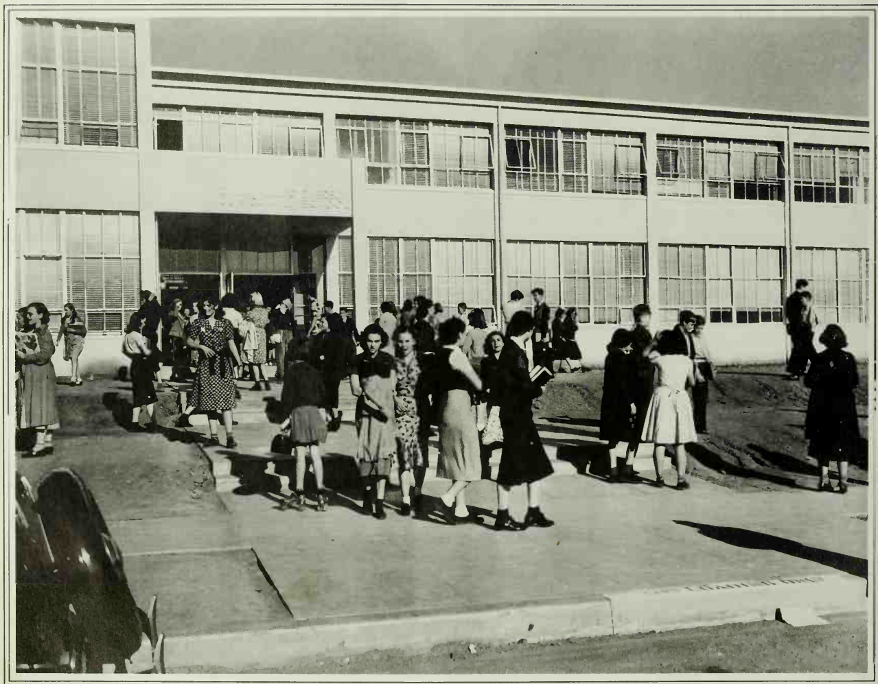
Milling students in front of newly-constructed Ralph Waldo Emerson Junior High School, Los Angeles, 1946. By 1953, when Gubser left California for the 83rd Congress in Washington, the need for more schools to service the post-World-War-II baby boom was critical; Gubser spent his term in Washington attempting to rectify that problem, with little success. CHS Library, San Francisco
