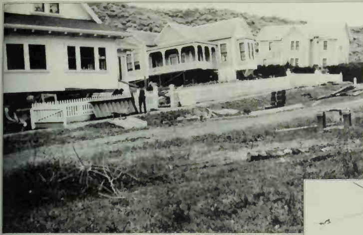
Houses toppled from their foundations, Bolinas, Marin County, April 1906. It is not well known that the great quake caused severe damage outside of San Francisco, particularly in lightly-settled Marin County and down the San Francisco Peninsula to San Jose. CHS Library, San Francisco
