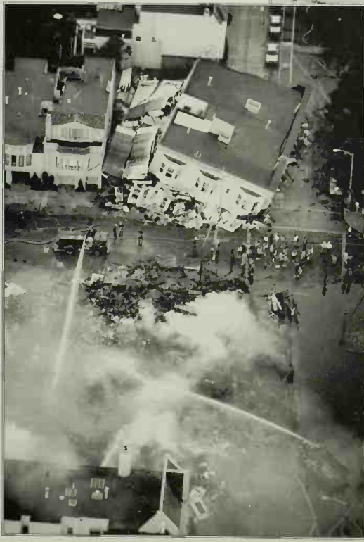
Marina District, San Francisco, after the earthquake of October 17, 1989. Photograph by Deanne Fitzmaurice. Courtesy San Francisco Chronicle
